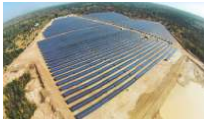
Thailand EPD 16MW Solar Power Station
