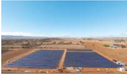
Australia Bungama 1.88MW Solar Power Station
