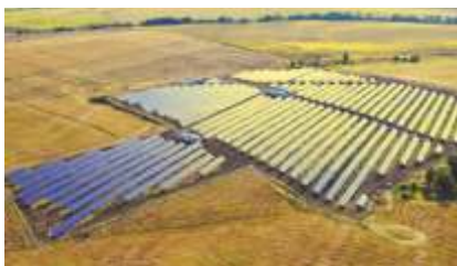
Smolnik 2.8MW Solar Power Station
