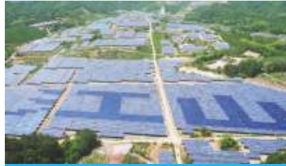
Jiangshan Agriculture Complimentary 200MW Solar Power Station
