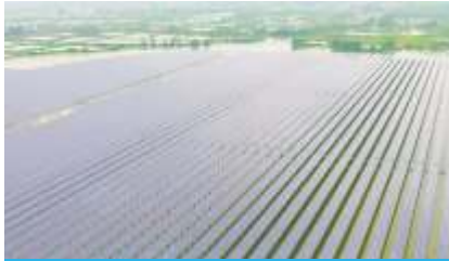
Huzhou Fishery Complementary 82MW Solar Power Station
