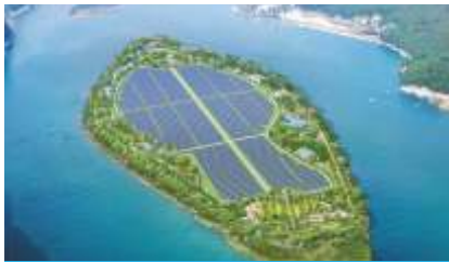
Korea Boongeo 9MW Solar Power Station
