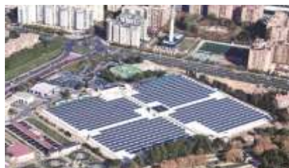
Spain Zaragoza 2.35MW Solar Power Station
