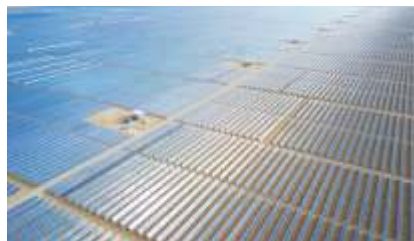
Saudi Arabia Sakaka 405MW Solar Power Station
