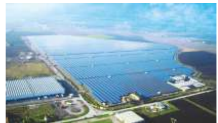
Rovigo 70MW Solar Power Station
