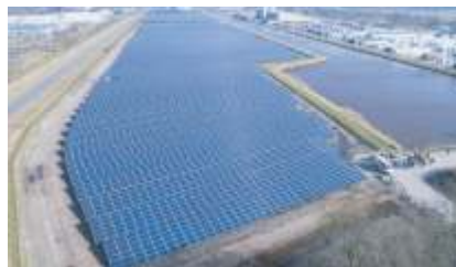
Netherlands Veendam 15.5MW Solar Power Station
